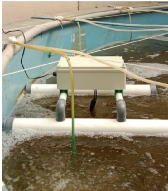
Fig. 1. Water quality sensor node made at BPBAP Situbondo
