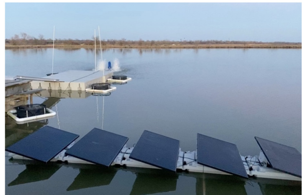
Figure 2: Pilot Floating Solar Aeration System at Texas A&M AgriLife Aquaculture Research and Training Facility
