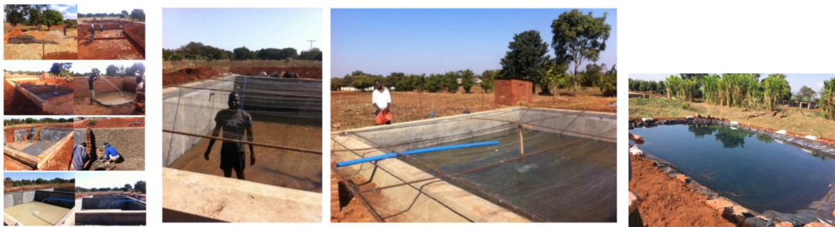
Construction of two types of fish ponds: concrete vs local plastic materials.
