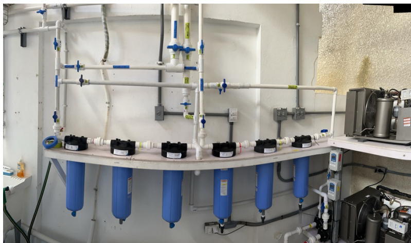
Figure 1. Filtration and chiller system at Puerto Rico, Naguabo Aquaculture Center
