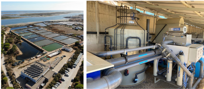
Figure 1 - Aerial view and RAS system on EPPO
